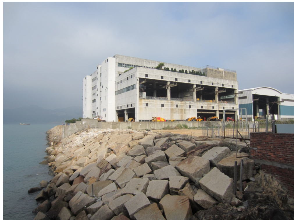
Photo 3 – Artificial Seawall in front of the cable landing point has been reinstated to its original conditions.
