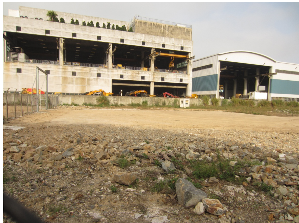
Photo 4 – Areas in vicinity of the cable landing point have been cleaned.
