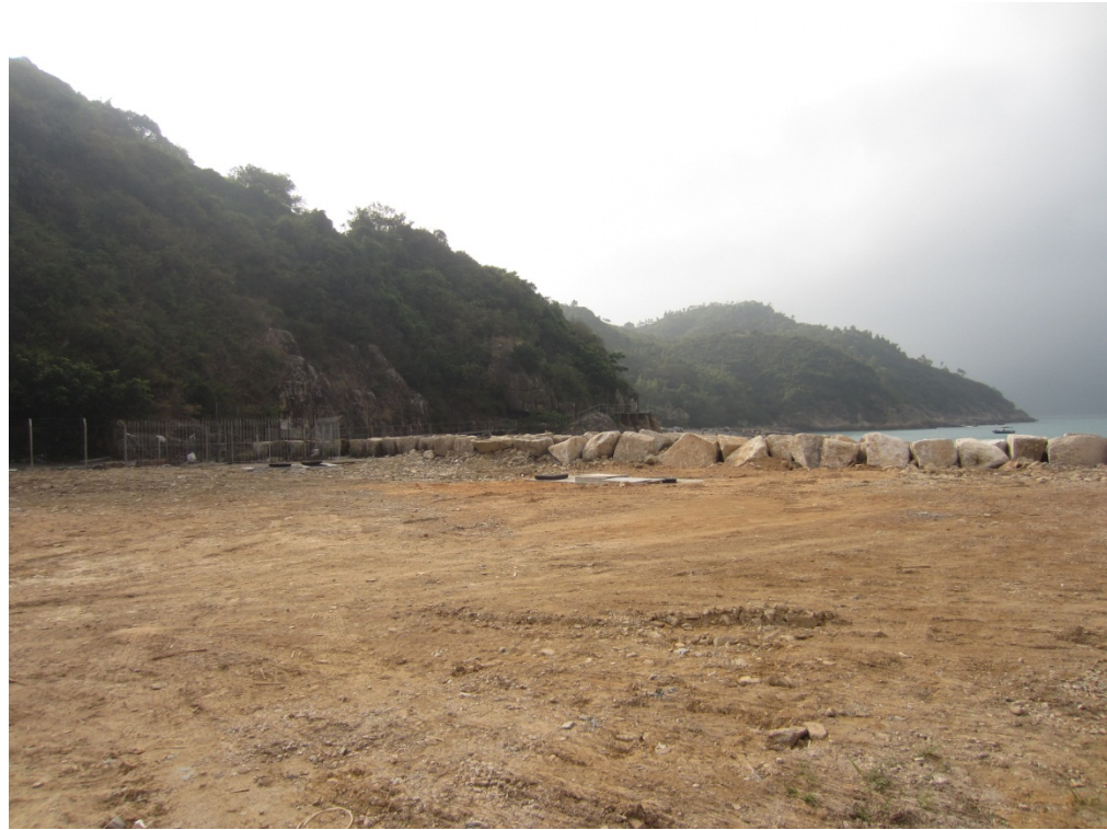
Photo 1 – Construction of the new beach manhole has been finished and the site has been reinstated to its original conditions.
