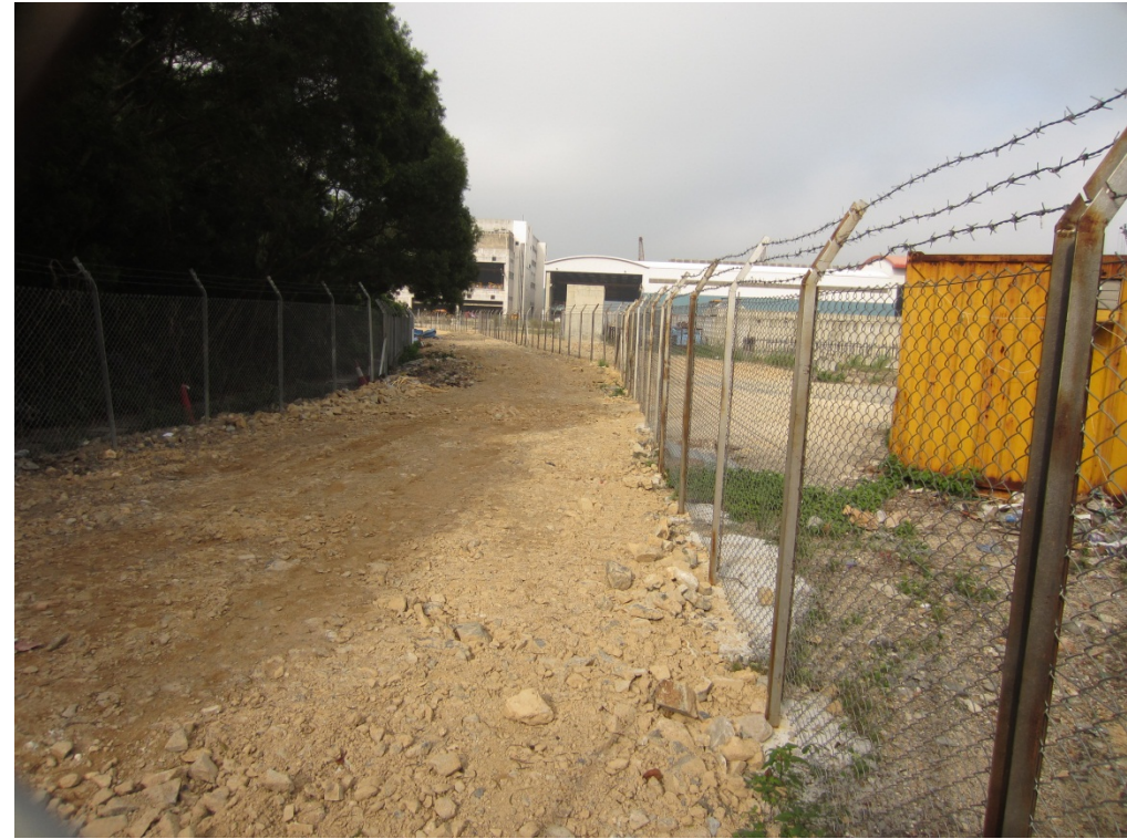
Photo 2 – Construction of the land duct has been finished and the site has been reinstated to its original conditions.
